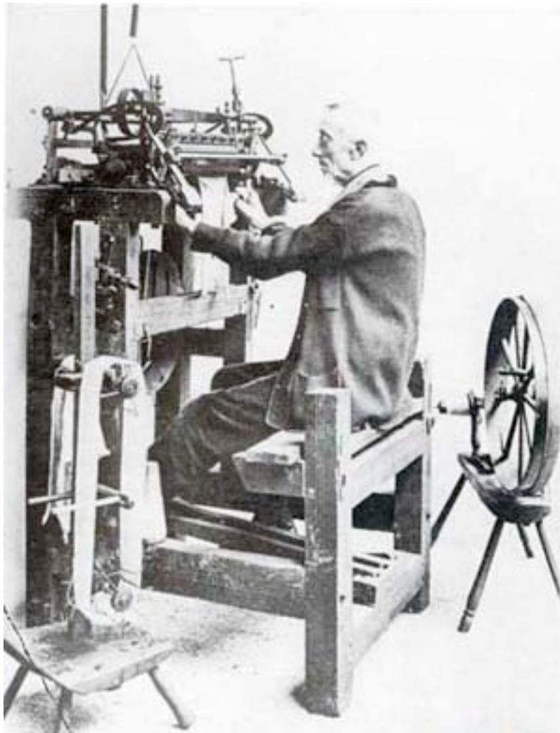
Figure 1. The First stocking frame knitting machine by William Lee in 1589 1 .
